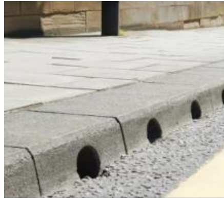
Figure 9. Drainage kerbs; source: [21]
