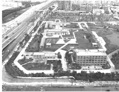
Figure 1. Zhuhai Qianshan Water Purification Plant
