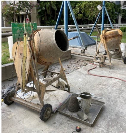
Figure 1. Mixing Concrete using Mechanical Concrete Mixer.
