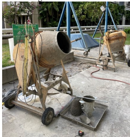
Figure 1. Mixing Concrete using Mechanical Concrete Mixer.
