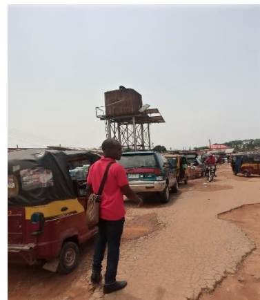
Figure 16. Water storage tank
