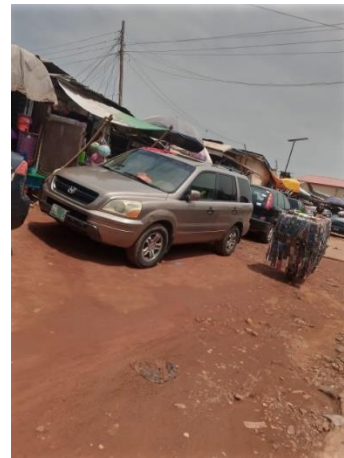
Figure 14. Image of the Derelict Road Network
